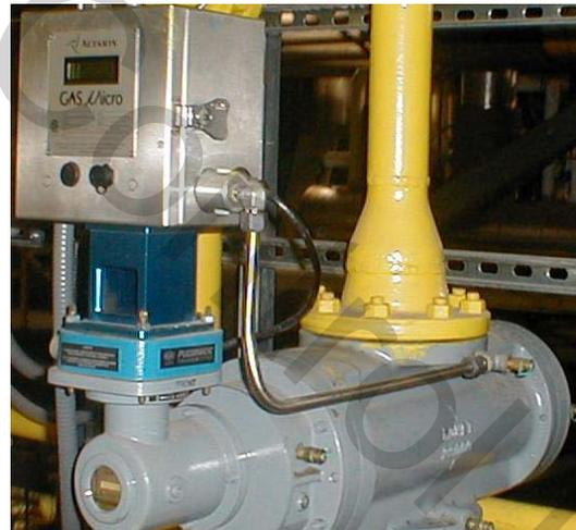
Pictured above: Rotary Meter with Pulser Installed Under the Galvanic PT Corrector
