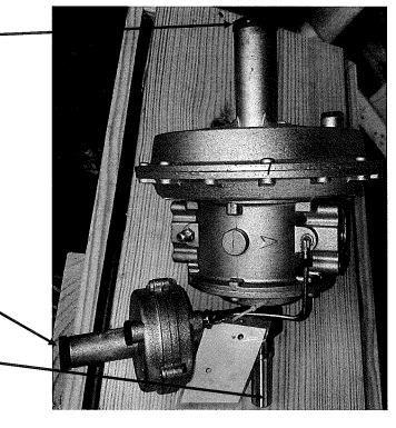
Installation Suggestions. Install straight "pipe" pieces on inlet and outlet with minimum length of 5 (five) time s diameter.
