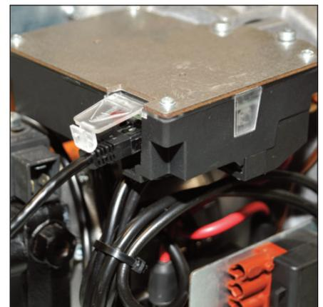
**!** The diagnostic tool includes connection cable with RJ45 connector. It has to be interfaced only with Ecoflam burners equipped with Thermowatt “E-BCU gas” or “E-BCU oil” control boxes. Before tool connection/disconnection switch off burner electric supply in order to injury to people or appliance.
